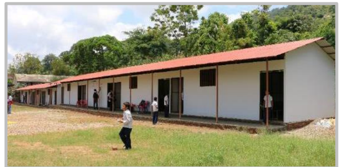
School Constructed by NYF at Gorkha
